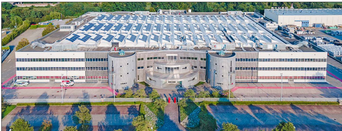
Elemaster's headquarters in Lomagna, north-east of Milan, Italy
