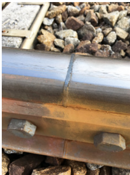
FIG. 6: Rail joints are specific points, which can be monitored via FTS by storing their base signature in a first place
