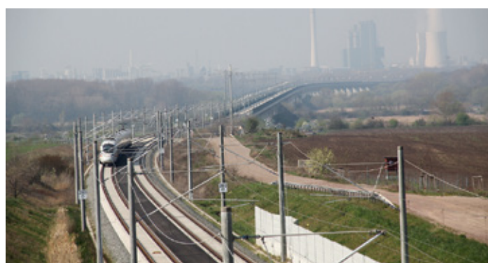
FIGURE 3: The Saale-Elster viaduct (Photo: DB AG/ Hannes Frank)
