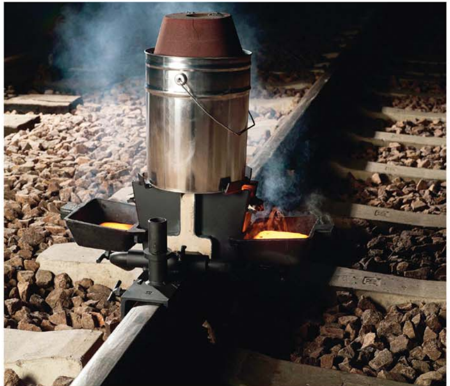
Thermit® welding process
